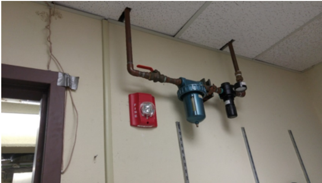
On: the red handle is turned 90 degrees.
